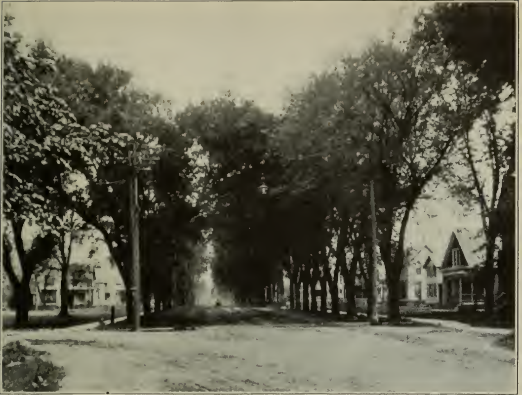
LOOKING ALONG SECOND STREET, ROCK FALLS
