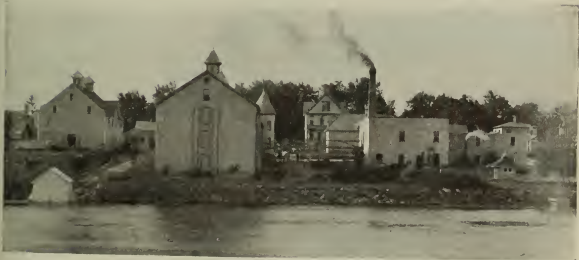
VIEW OF HOARD'S CREAMERIES, FORT ATKINSON, FROM THE RIVER
