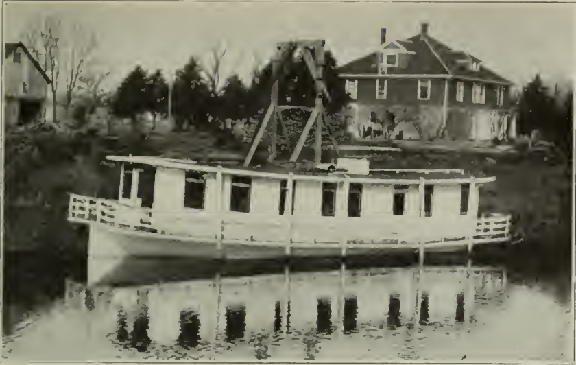
OPENING OF THE HENNEPIN CANAL AT ROCK FALLS, 1907 Government boat "Rambler" enters the locks
