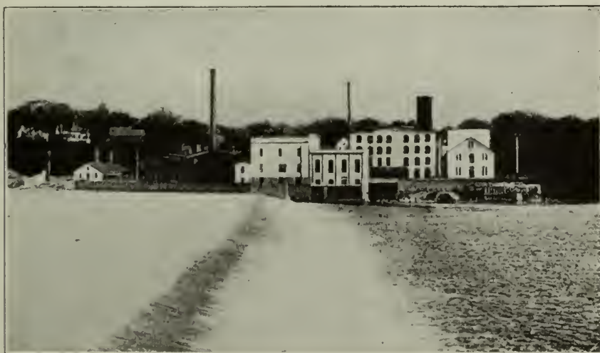
DAM AND POWER HOUSE, DIXON
