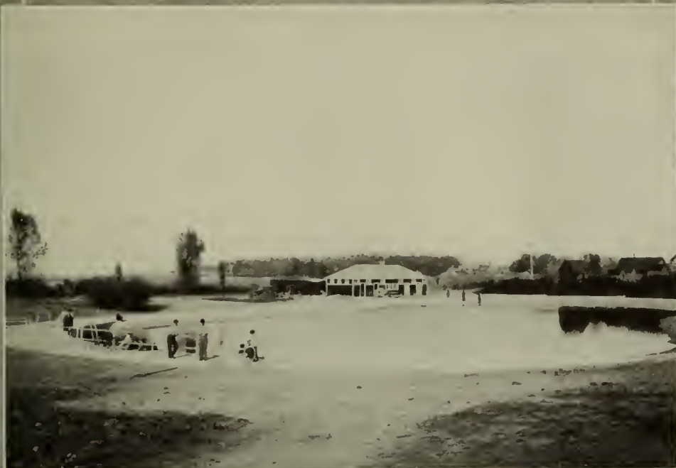
Looking north showing swimming pool
