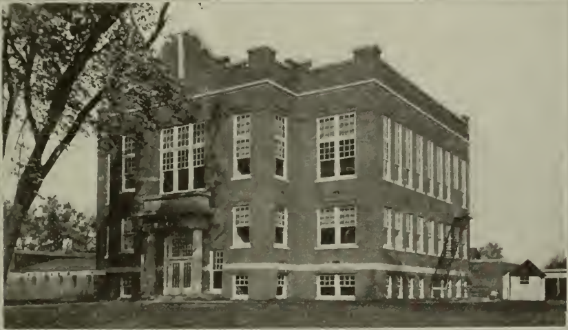
Weathersfield High School
